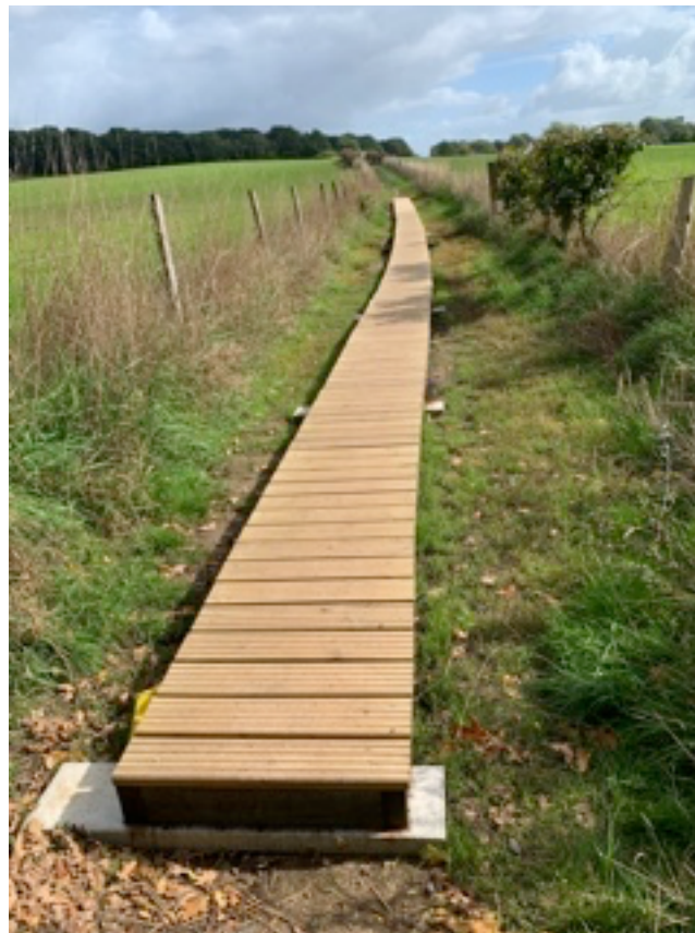
Our new causeway on the 'Roman Road' footpath. Ditchling
