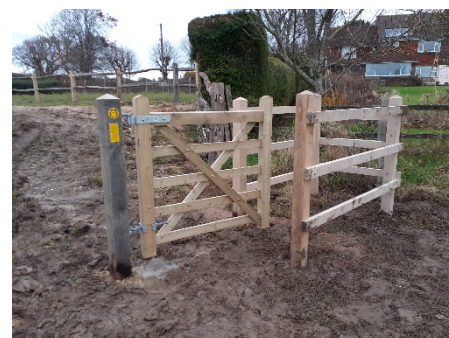
A new MG "Kissing Gate" being installed at start of a re-routed path
