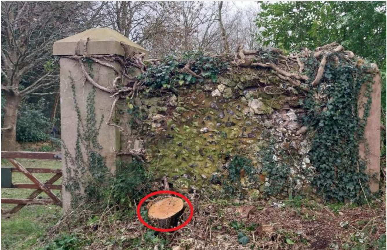
Photograph 1 – Showing Tree Removed from East Side of Flint Wall
