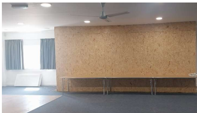
Temporary Hoarding, Court Bushes Function Room
