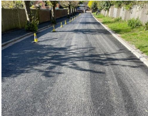
South Avenue Resurfacing
